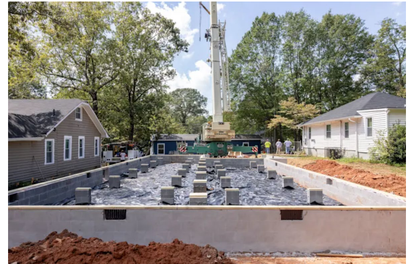
Set on masonry foundation
